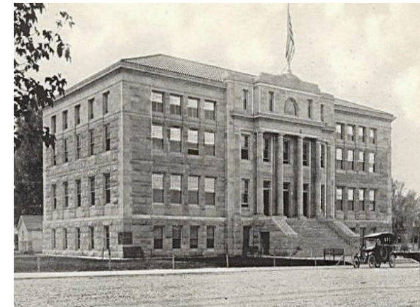
Montrose County Courthouse in the mid 1920's
